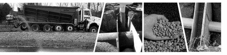
AquaBlok<sup>®</sup> is a patented material based on a proven bentonite composite-aggregate technology. The use of a bentonite coating layer provides a low-permeabiliy sealing layer for sediment remediation and in a range of upland and aquatic sealing applications.
